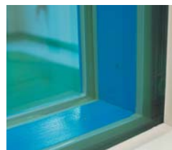
Dual structure window consisting of bulletproof glass and fireproof glass
